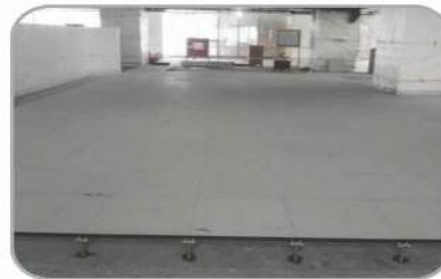
Al Rajhi Bank Head Quarters - Riyadh Calcium Sulphate Panels Raised Floor Installation
