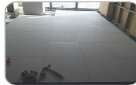
Al Rajhi Bank Head Quarters - Riyadh Calcium Sulphate Panels Raised Floor Installation
