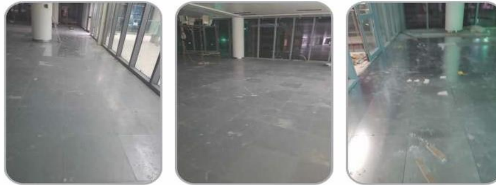
Saudi Electrical City Company Head Quarters Riyadh Lindner Wood Core panels Installation
